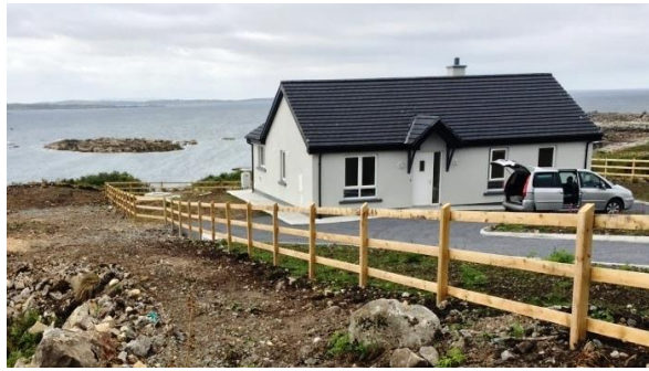
Single Rural dwelling at Cill Chiaráin, Conamara
