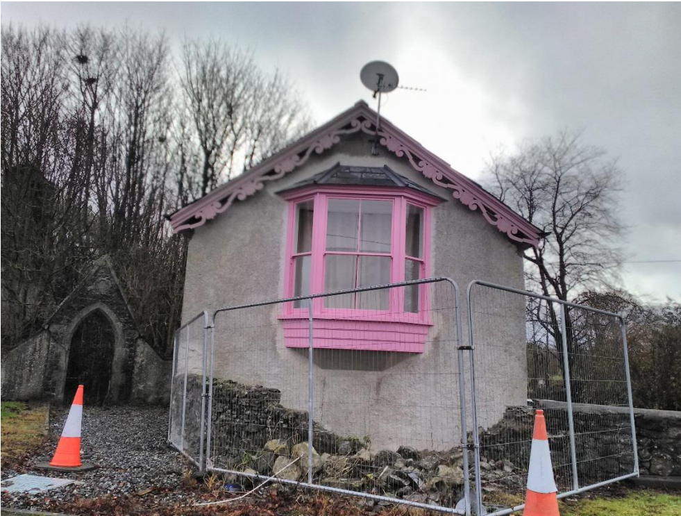
Park Cottage Eyrecourt - Repairs to bay window and surrounding lime render
