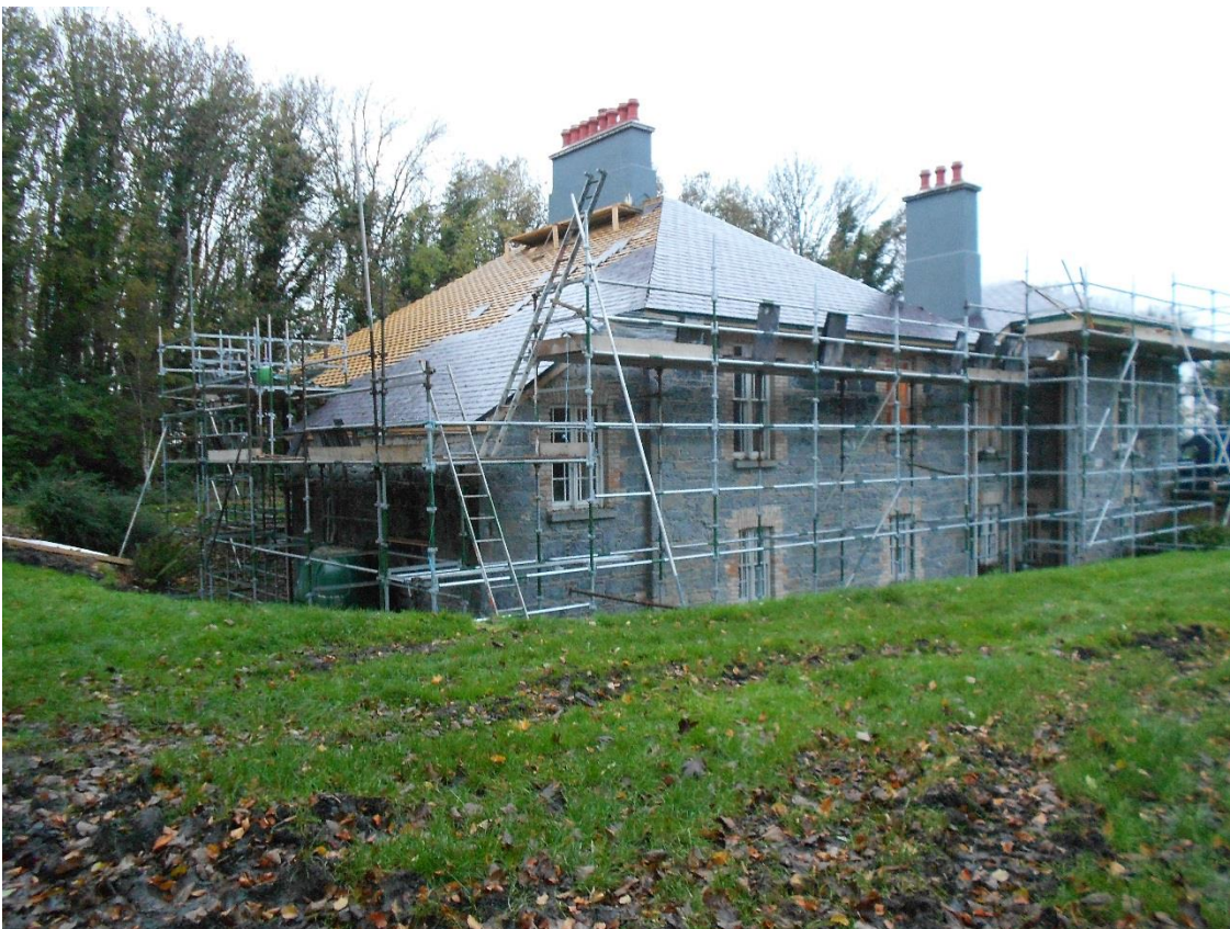
Rathville House, repairs to roof and chimneys
