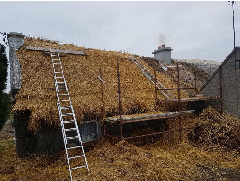
Straw thatch coat underway at Moyower, Eyrecourt
