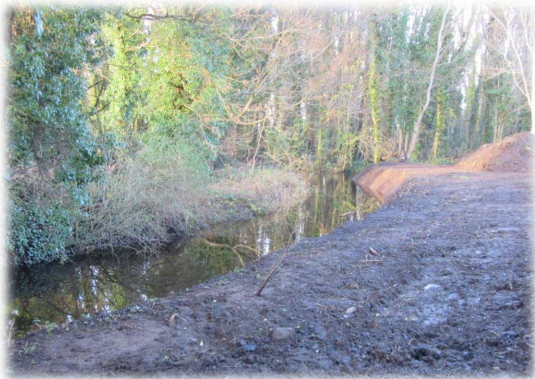
South Galway, Gort Lowlands Flood Relief Scheme – Channel clearance works at Roxborough swallow holes undertaken as advanced works on the scheme
