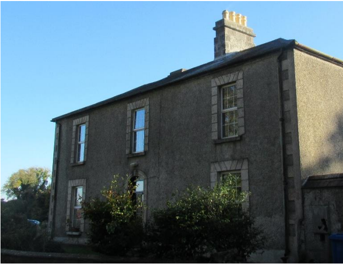
Cartron House, Aughrim - Repairs to chimney
