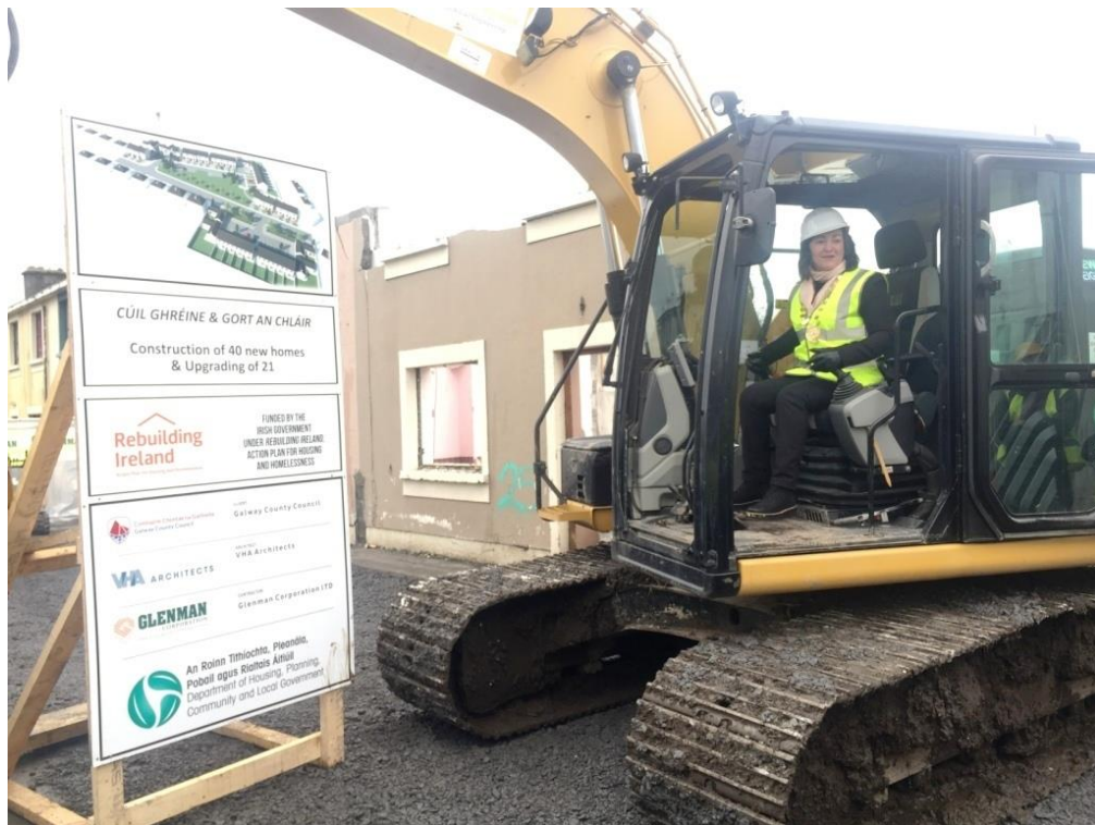
An Cathaoirleach Cllr. Eileen Mannion at the sod turning of the development of Cúil Ghréine and Gort an Chláir, Tuam.
