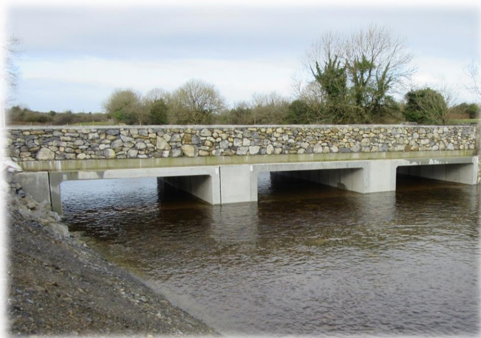
Dunkellin River & Aggard Stream Flood Relief Scheme – Newly installed flood eyes at Rinn Bridge in operation
