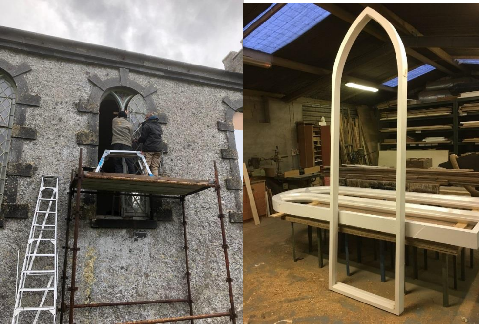
Ardrahan Church - Repairs to windows
