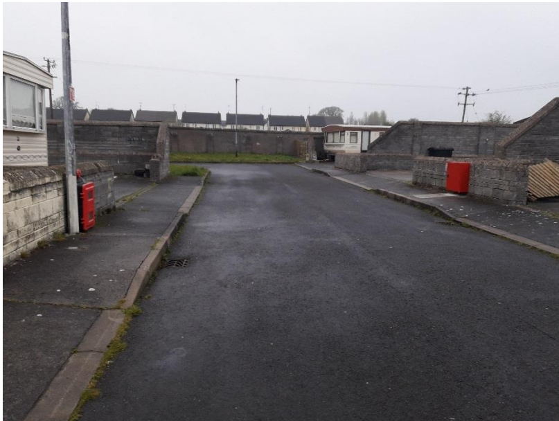
Upgraded access road to Tuam Halting Site
